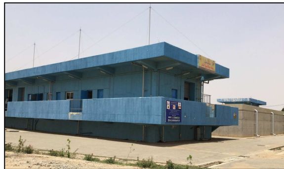
Mahta Water Treatment Plant 1
