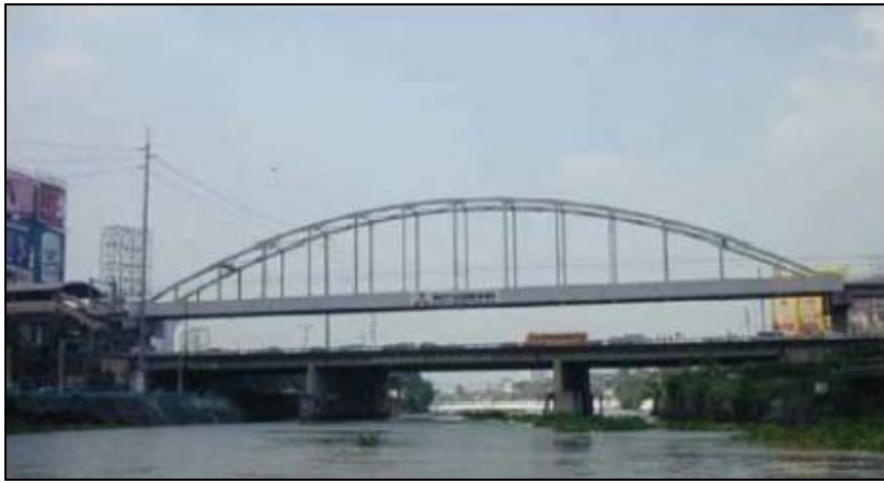
The Guadalupe Bridge along the Epifanio Delos Santos Avenue (EDSA) in Metro Manila is one of the seven (7) priority bridges proposed for retrofitting / replacement identified under this Project. The plan for the bridge is now included in the Loan Agreement for the Metro Manila Priority Bridges Seismic Improvement Project between the Republic of the Philippines and JICA.
