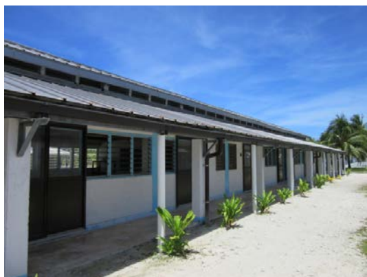
Rehabilitated Special Classroom Block
