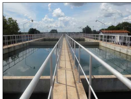
Concepcion Water Treatment Plant: Chemical Sedimentation Tank
