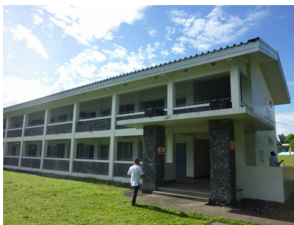
Schools Designated as Evacuation Shelters Developed under This Project (Sto. Domingo Central Elementary School)
