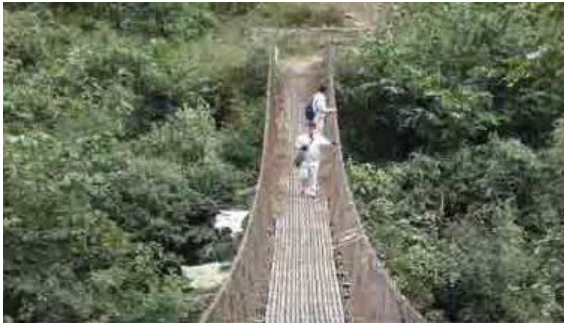
(Before the construction: Former Jangbi Bridge)
