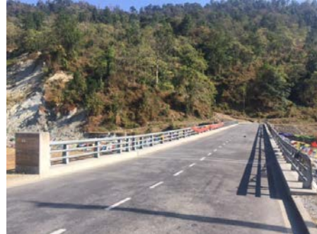
(After the construction: Jigmeling Bridge)
