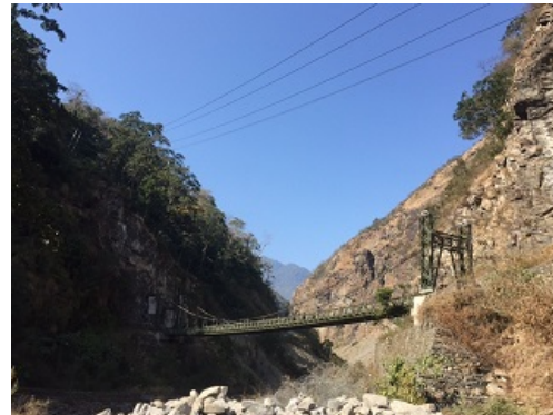
Reotala (Mangdechhu) Bridge 1 constructed in the mountain
