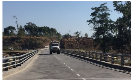
(After the construction: Dolkhola Bridge)
