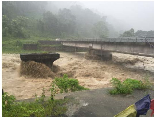
Jigmeling Bridge at a time of flooding of the river (The foreground is a pier of the old bridge: Photo provided by a local resident)
