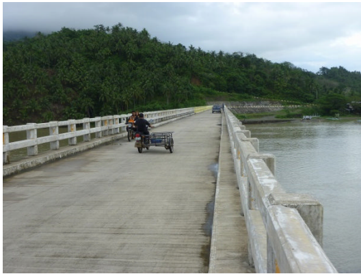
Photo 3: Road Surface of the Umiray Bridge
