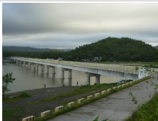
Constructed Umiray Bridge and Access Road
