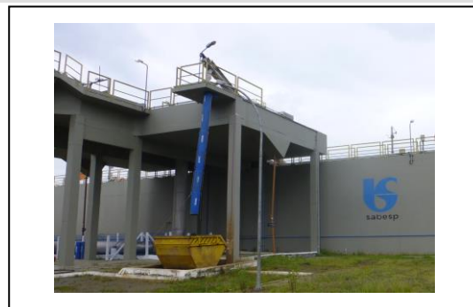
A new wastewater treatment plant in Itanhaém
