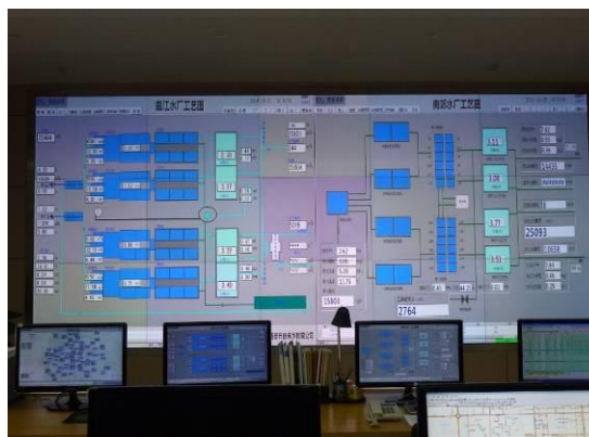
Central Control Room
