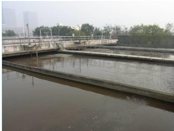
Biological Reaction Reservoirs at the Sewage Treatment Plant in the Southwestern Suburb of Xi'an City
