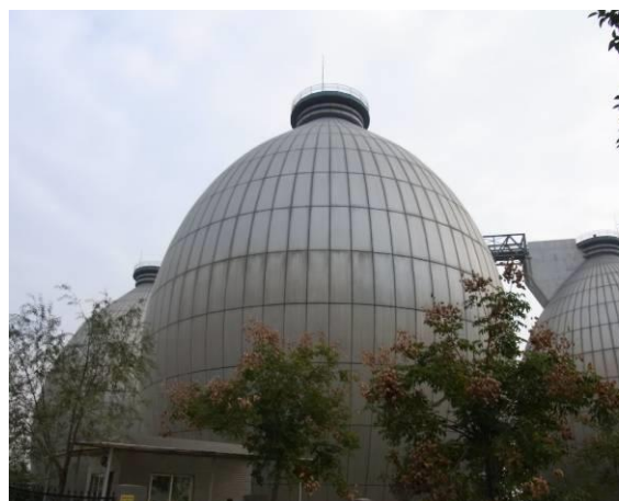
Sludge Digestion Tank at the Xi'an Yuanle Village Sewage Treatment Plant
