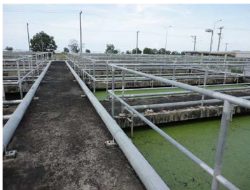
Waste Water Treatment Plant
