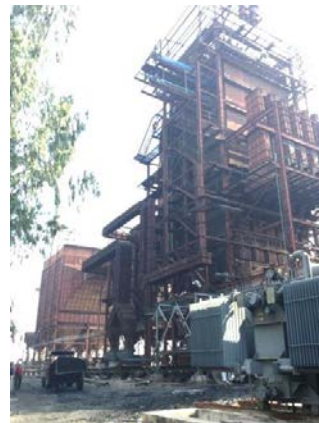
Company A: Outside View of the Power Generation Facilities
