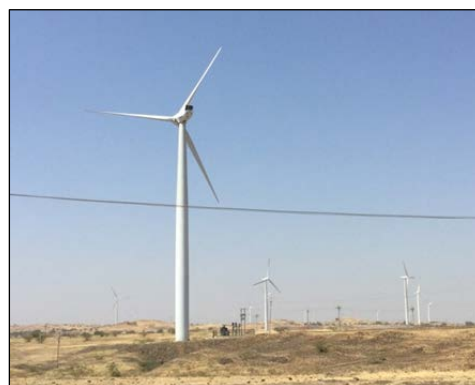
Wind power generation financed by the project
