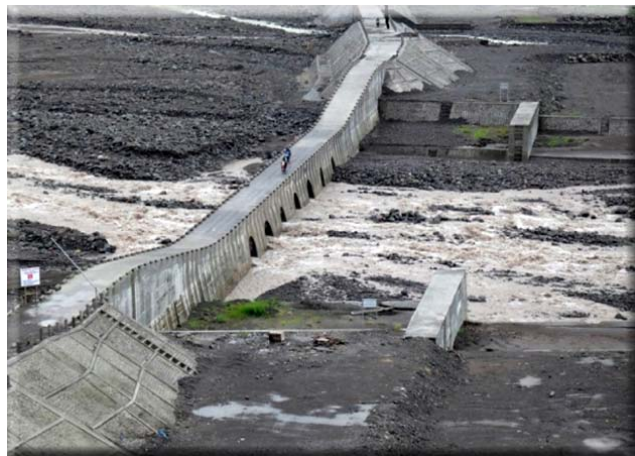
(Consolidation Dam : Mt. Bawakaraeng Component)
