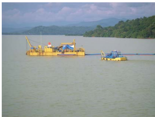
Dredging Works near the Water Intake of Bili-Bili Dam
