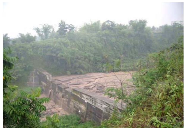
Arrested Debris Flow by Sabo Dam at Krasak River (Source: Material provided by Executing Agency)
