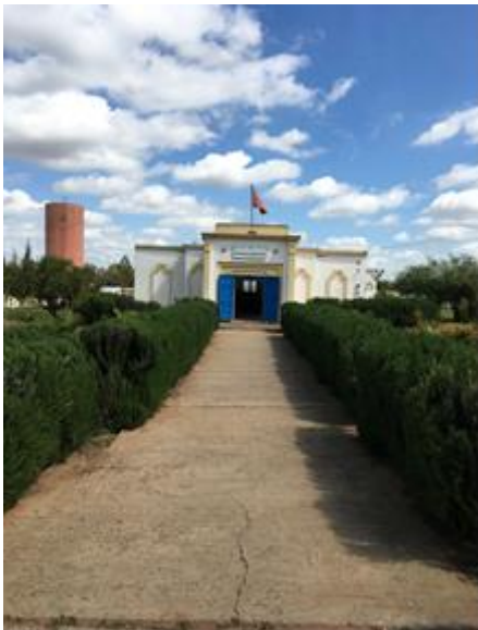
Health center near the road
