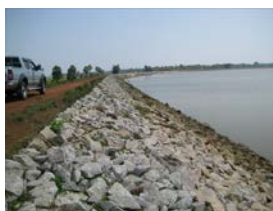
Tank Bund in Batticaloa District, Eastern Province (Kadukamunai Kulam Irrigation Scheme)
