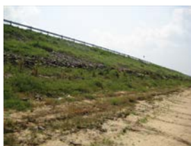
Tank Bund in Ampara District, Eastern Province (Namal Oya Irrigation Scheme)
