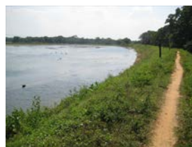
Tank Bund in Polonnaruwa District, North Central Province (Kambukunawale Irrigation Scheme)
