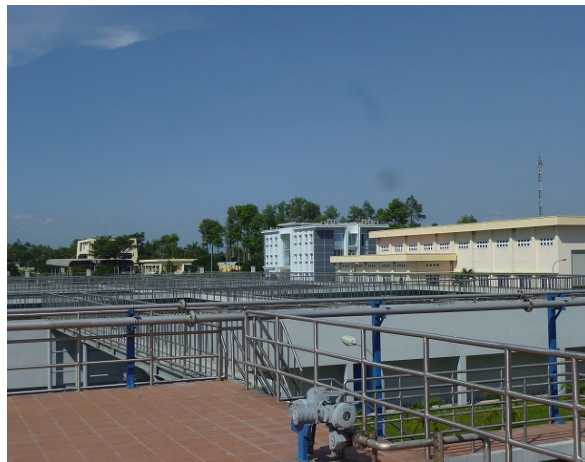
Constructed Water Treatment Plant in Dong Nai Province
