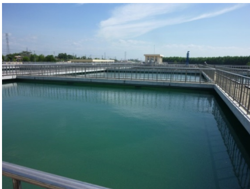
Photo 1: Constructed Water Treatment Plant in Dong Nai Province
