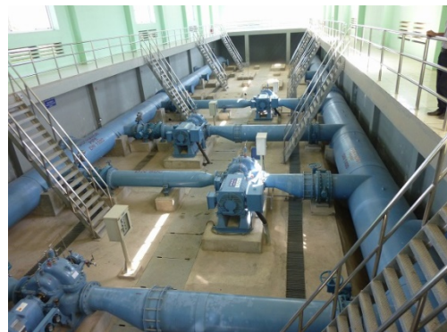
Photo 2: Constructed Water Pumping Station in Dong Nai Province
