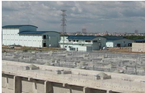
Binh Hung Wastewater Treatment Plant
