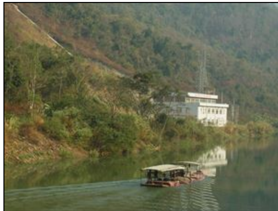
Hydropower Plant in Nghe An Province
