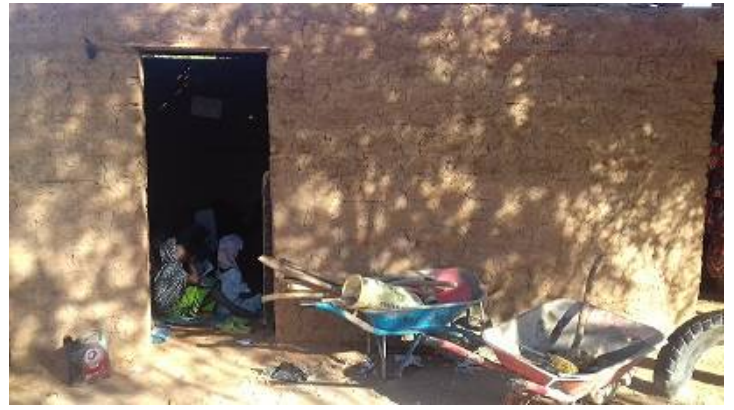
Classroom constructed by CGDES
