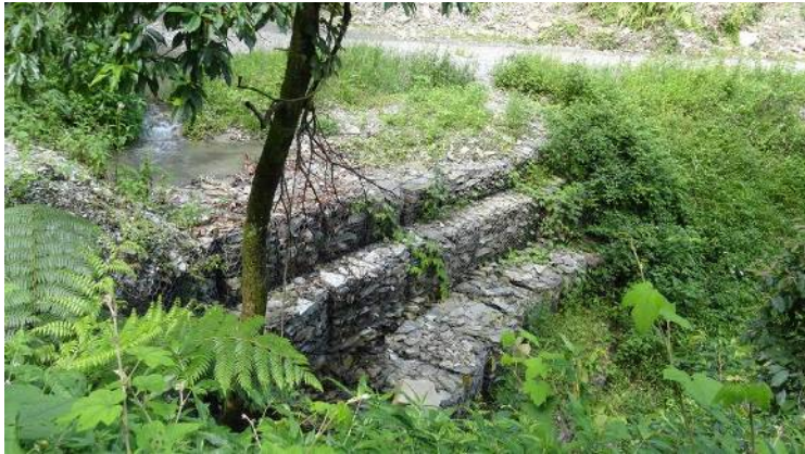
Gully control to protect motorable road at Dhital, Kaski district
