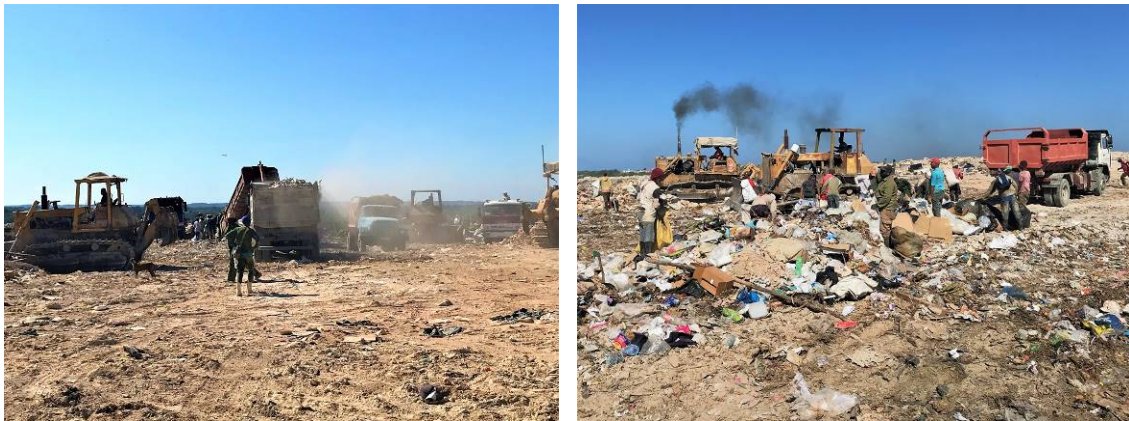
Calle 100 disposal site soil covering (left); waste pickers operating in the waste dumping zone (right)
