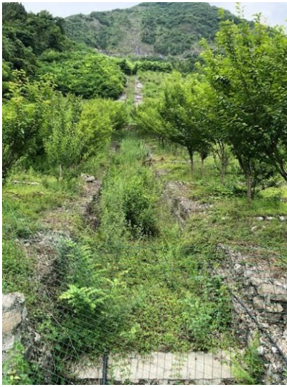
Test construction site of the project in Beichuan County
