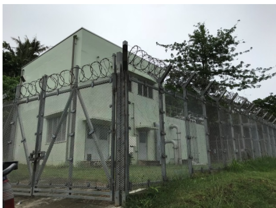
Fence built through the project (Borderline Pump Station)
