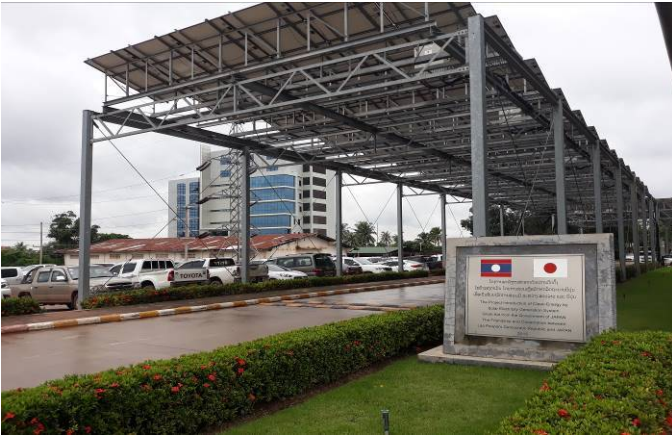
(PV system at EDL building)
