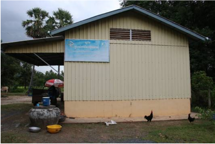
Warehouse of Phnom Touch Samaki SGG to store the produced seed (Banan District, Battambang Province)
