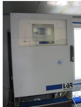
The toxic sensor installed in the upper stream area of Heihejinpen Dam Lake. No failure occurred since installment.
