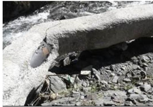
Photo 5. Damage to protective cover of transmission mains at Namly Mira intake facility due to flooding
