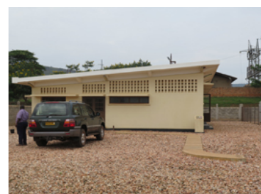
Substation Building (Rwinkwavu)
