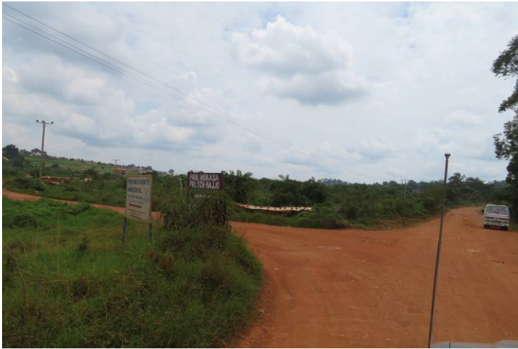
One of the district roads in Mukono district
