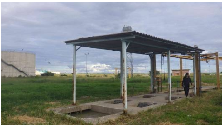
Grid Chamber, Zengeza Sewage Treatment Plant
