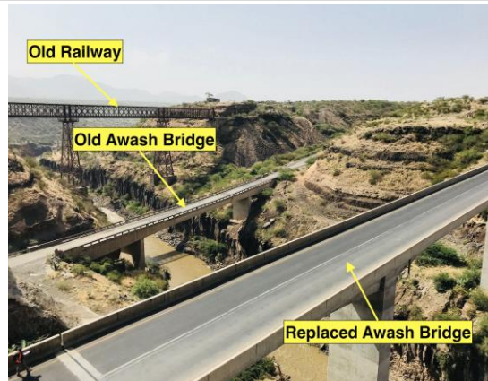
The Bridge Replaced by the Project 2
