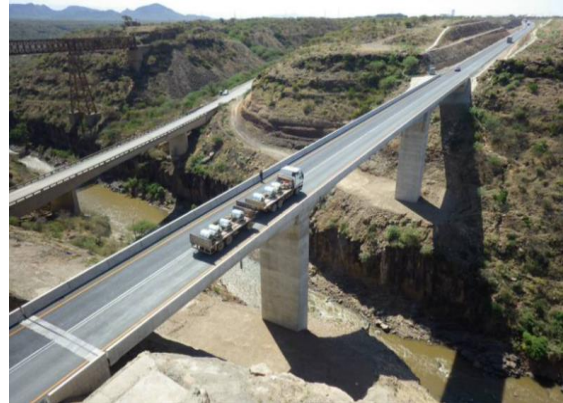
After the Construction 16
