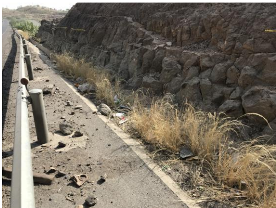
Photo 1: Drainage Facilities Covered with Sediment and Garbage
