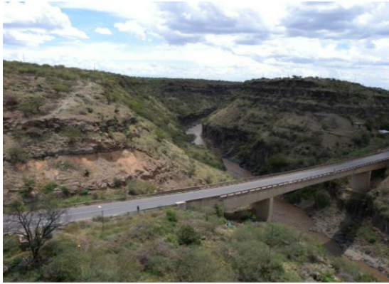
Before the Construction 15
