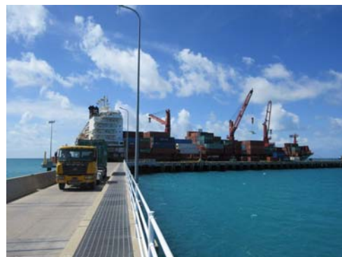
Wharf and Access Trestle Developed in This Project
