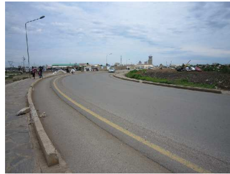
Part of constructed road
