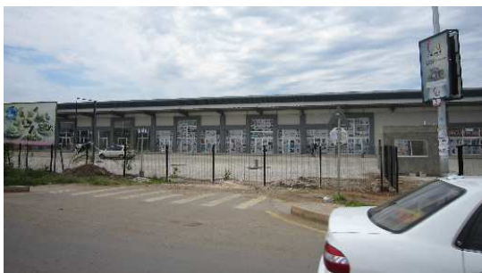
Photo: Shopping mall under construction along the road
