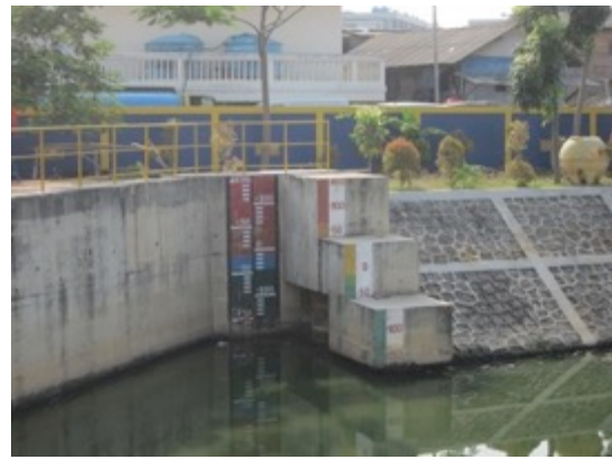
Photo 4: Pluit Pump Station The reservoir water level is visually monitored
