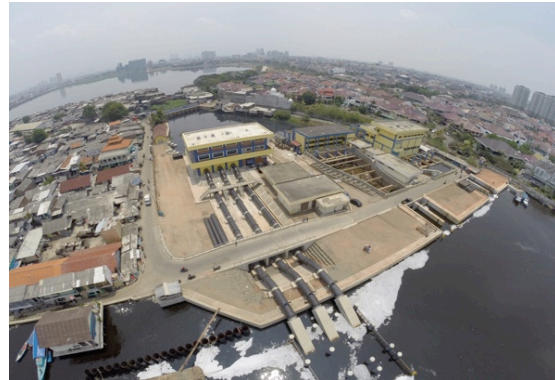
East Pump Station of Pluit after reconstruction 2
