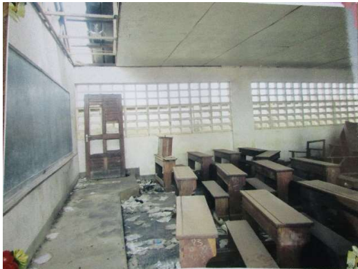
Photo 1. A Classroom Damaged by Arson
