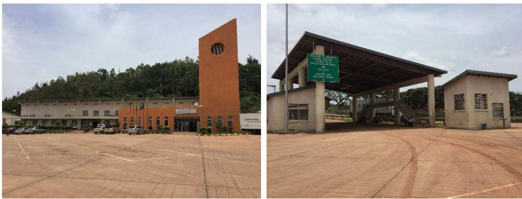
Photo 1. OSBP Facilities–Administration Building Photo 2. OSBP Facilities–Control Shed, Guard House
