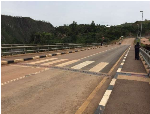
Rusumo Bridge Built by the Project
