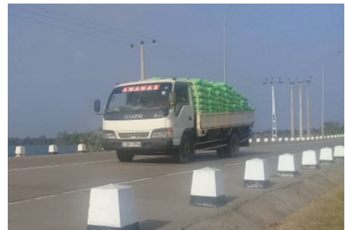
Photo 2: The opening of the bridge contributed to reducing truck delivery time and cost
