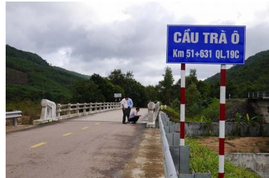
Trao O Bridge At the time of Ex-post Evaluation (2017)
