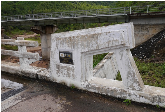
Tra O Bridge with repainting
