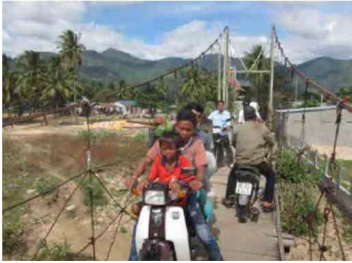
Tam Ngan Bridge, At the time of Planning of Phase III (2011)
