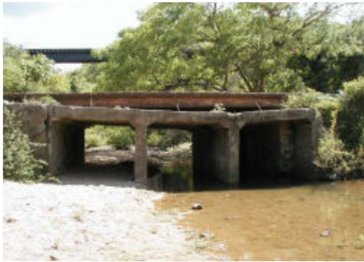
Trao O Bridge, At the time of Planning (2001)
