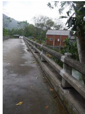
Khe Duong Bridge with repaired guardrails
