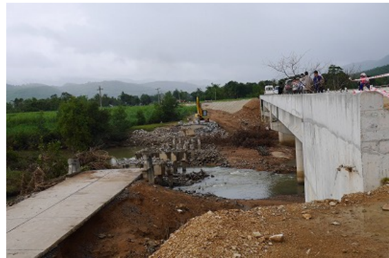
New and Old Tra Buong Bridge (Left is the bridge by this project)
