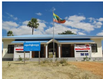
Newly-constructed Lat Seil RHC (at Ex-post Evaluation)
