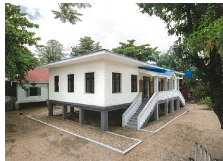
Appearance of a newly-constructed RHC (Raised-floor type)
