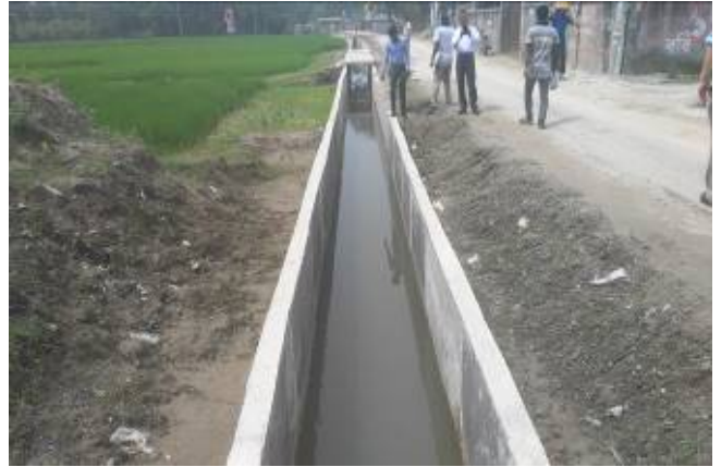
Drainage improvement in Rangpur (RCC)
