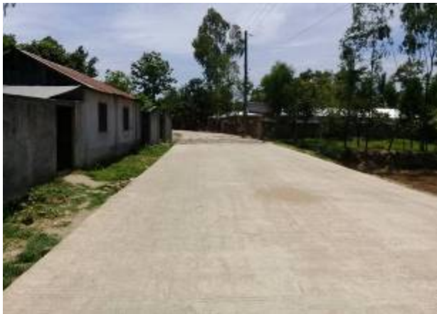
Road infrastructure Subproject in Gazipur (GCC)
