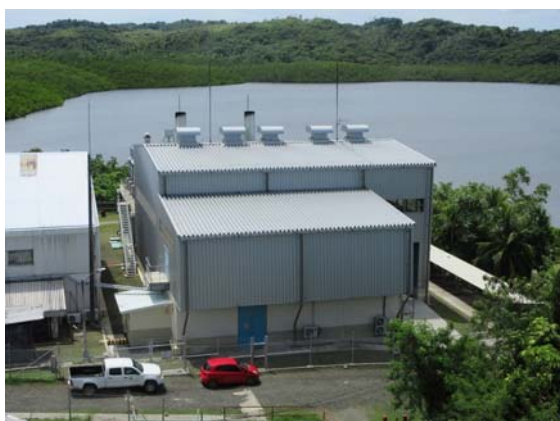
Panoramic View of the Power House
