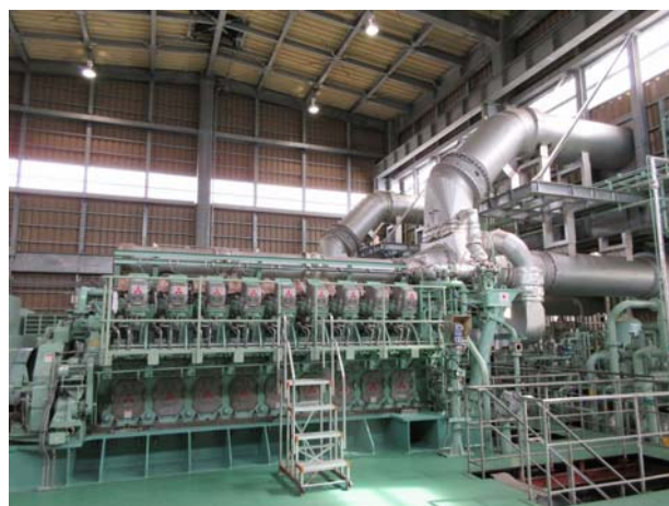
Generator Installed in this Project
