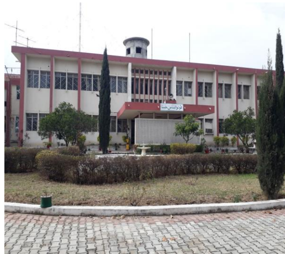
Faqirabad Transmitting Station
