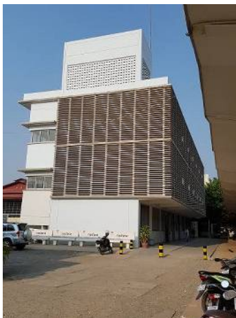
An exterior view of Lab Building
