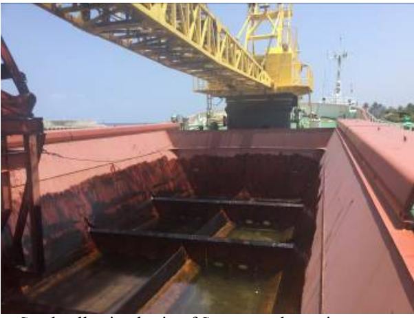
Sand collection basin of Sayuru under maintenance
