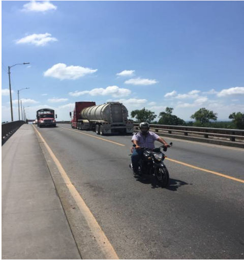
Commercial traffic going through the bridge
