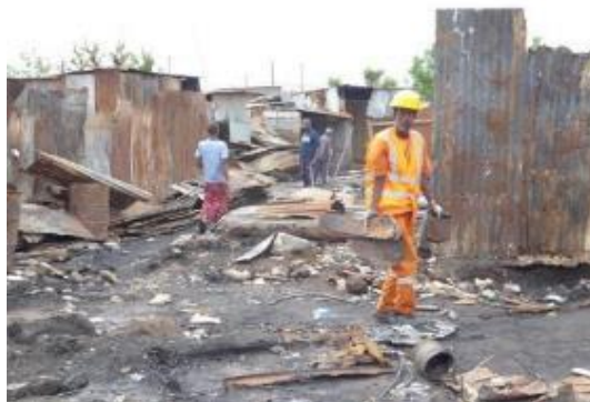
Fire debris clean-up of 26 houses in a densely populated area
