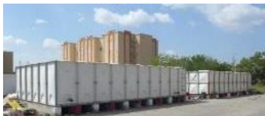
A water tank in the Sans-fil Fire Station
