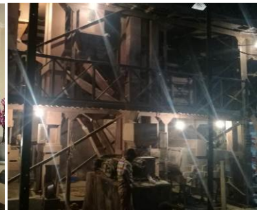
Milling factory where electricity is indispensable (Sylhet)
