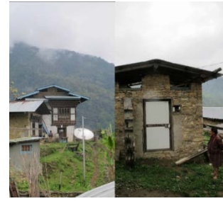
Photo 4: Langthel Gewog, Trongsa Dzongkhag Left: House electrified by the Project Right: Storage for Potatoes, where temperature is controlled by the electricity supply
