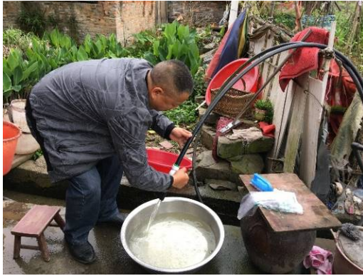
A drinking water facility installed at home
