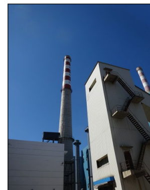
Southeast heat source plant: Chimney for dust collection and desulfurization (Hohhot Chengfa Development & Management Co., Ltd)
