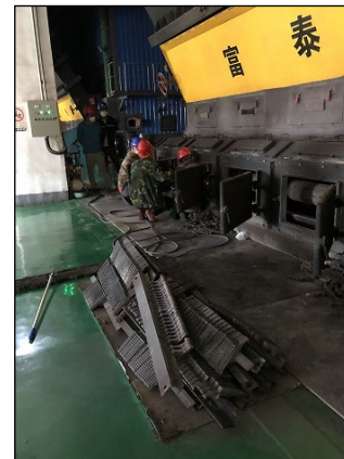
Bayan heat source plant: Boiler maintenance (Hohhot Futai Heating Supply Co., Ltd.)
