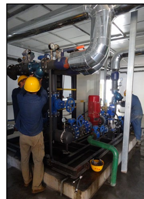
Maintenance of a heat exchange station (Hohhot Chengfa Development & Management Co., Ltd)
