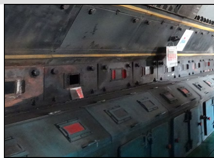
Boiler at Xinjiaying Power Plant B (Hohhot Chengfa Development & Management Co., Ltd)
