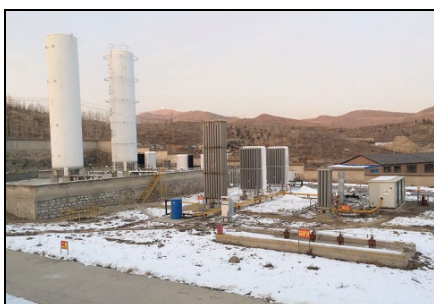
City Gas Project (Altay City)
