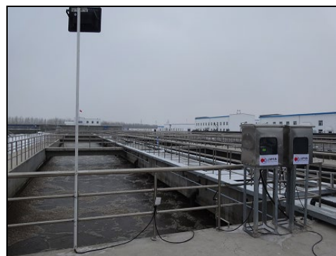
Kuitun Sewage Treatment Plant (activated sludge tank)
